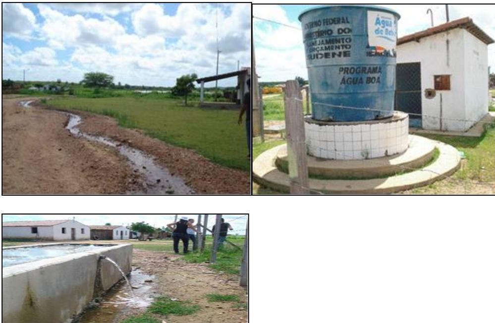
Figure 1. Salt water treatment station and disposal of saline waste in soil and water course
